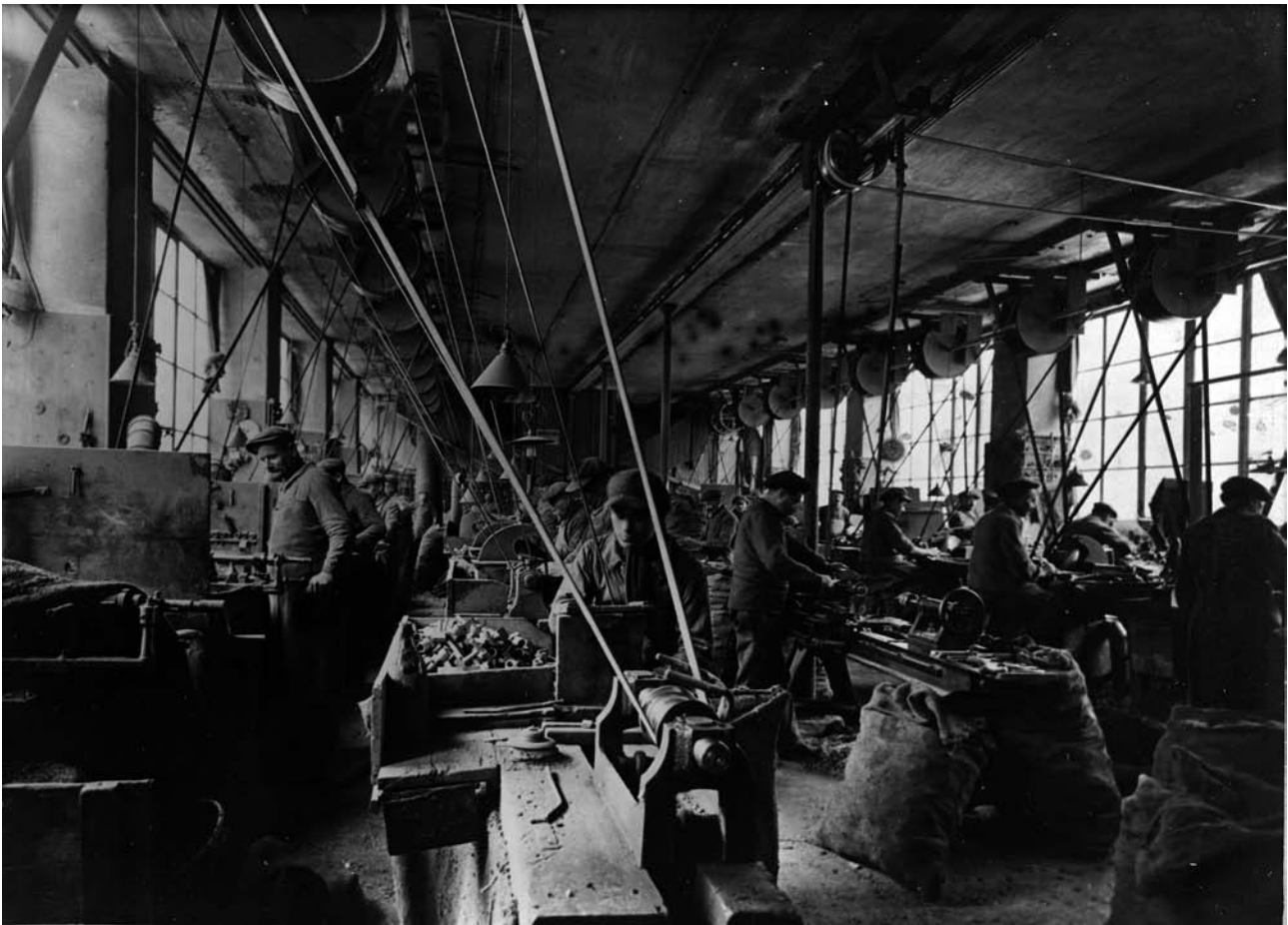
Figure 7: Belt driven lathes turning bowls at the La Bruyère factory c1920 (photograph courtesy of the John Adler Archive).
